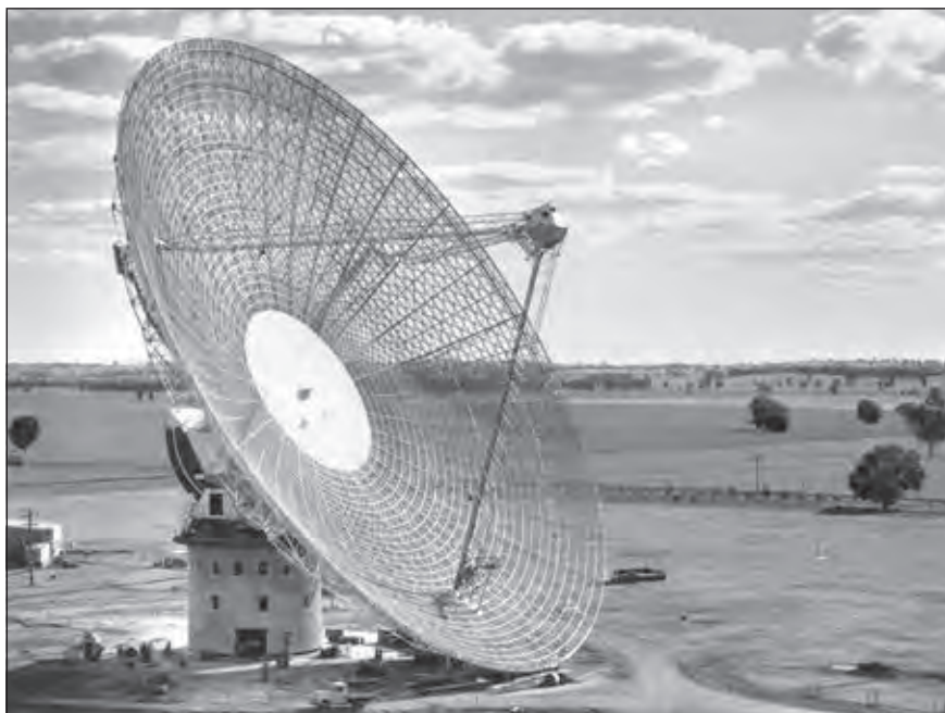
Parabolic radio telescope with a diameter of 64 m, second largest movable telescope in the world, in 1987 extended to 70 m, Parkes, 1961 (MÚA, A AV ČR, Luboš Perek collection, photo catalogue No. 507)
