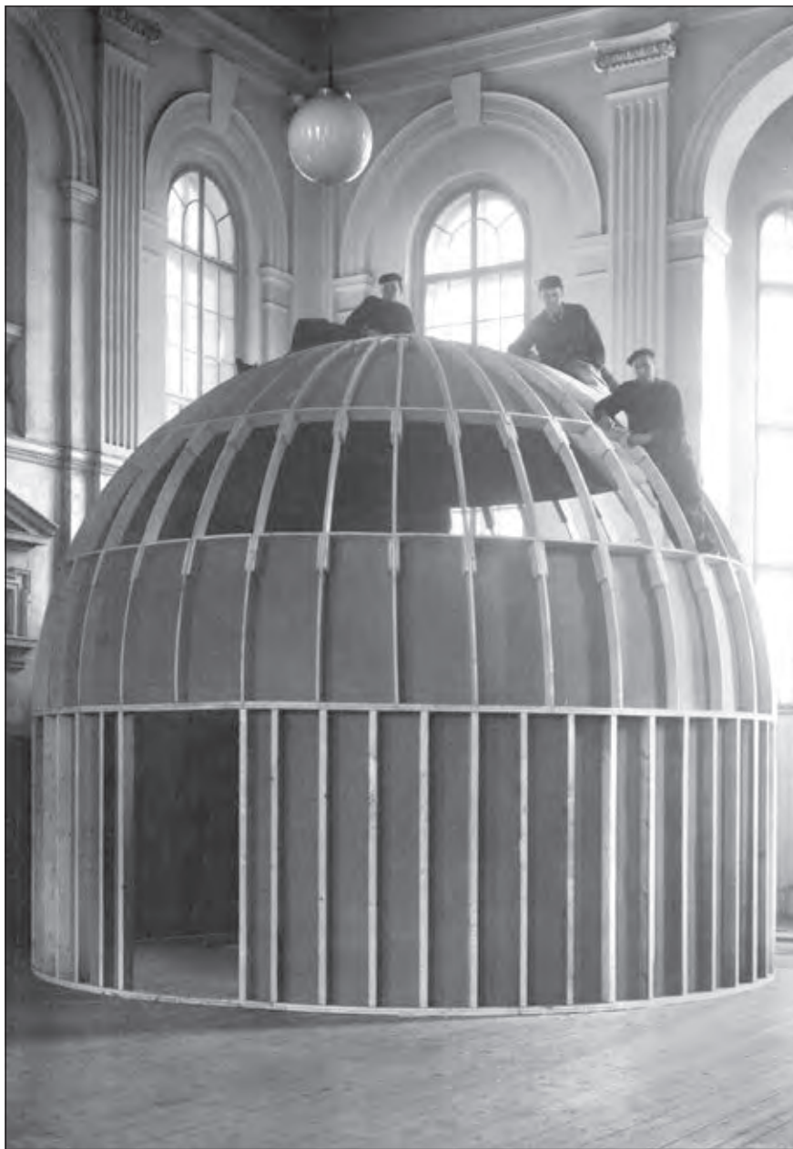
Construction of the dome for the school planetarium Nad Hamburkem, 1958 ( Hvězdárna a planetárium Plzeň collection )
