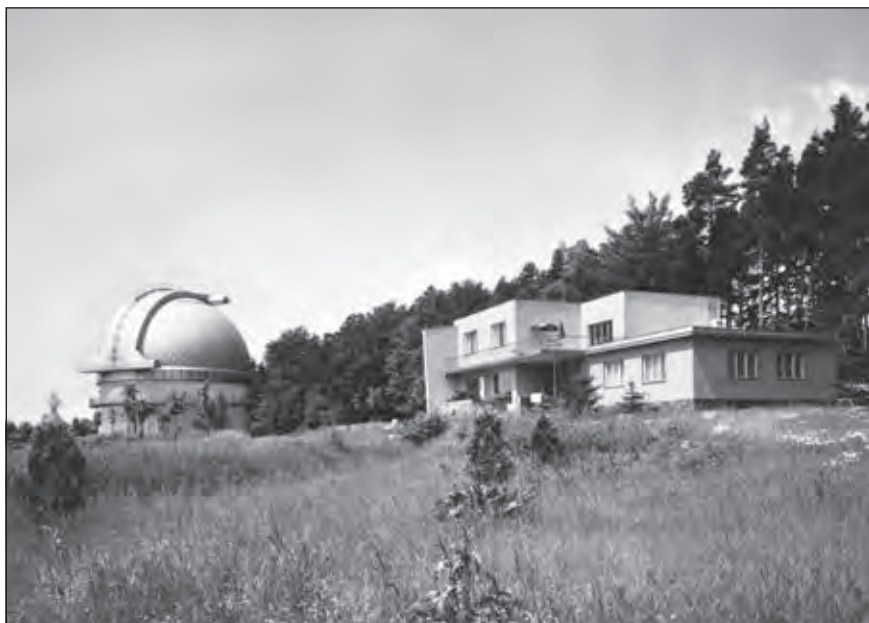
Perspective view of the dome of the two-meter telescope
